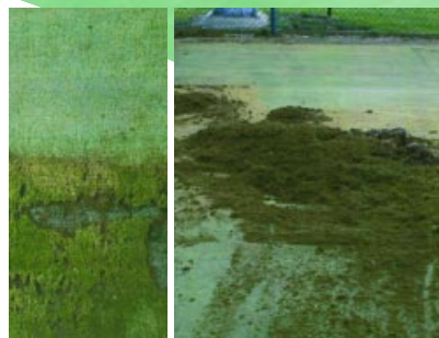
Build up of moss and contaminated sand
